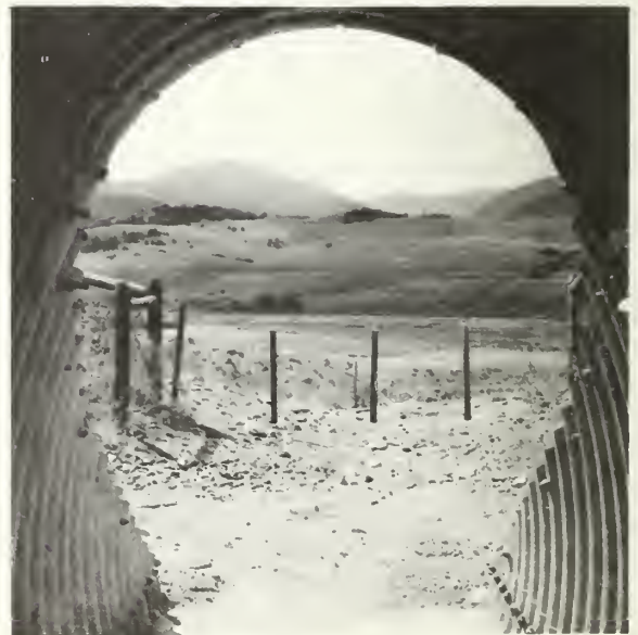
Looking West from WEST ENTRANCE
